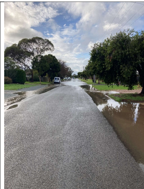
Photograph 1 – View east down Church St towards Fowler St
