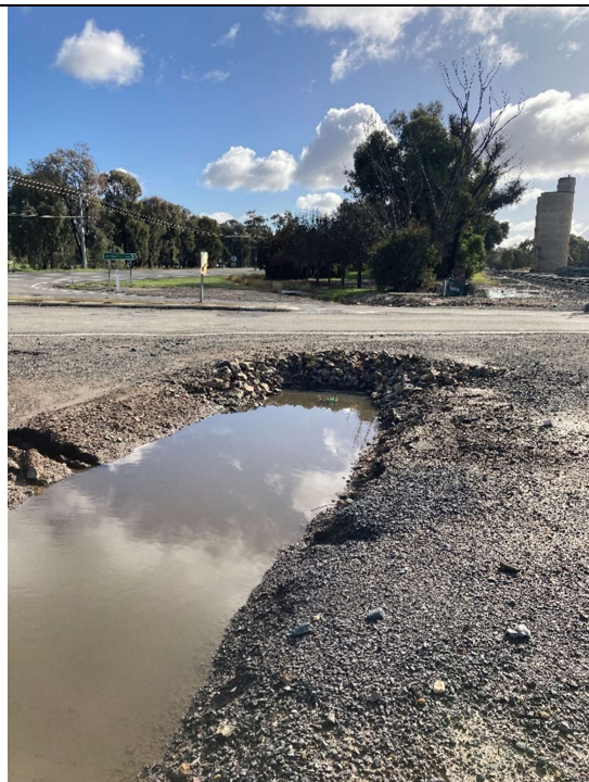
Photograph 3 – GV Highway roadside drain at Victoria Street, looking north
